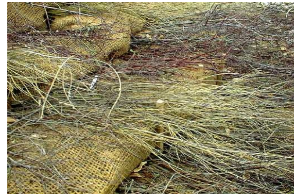
Photo 24. Brush layering with soil wrap, Raleigh, NC. Source: KCI
