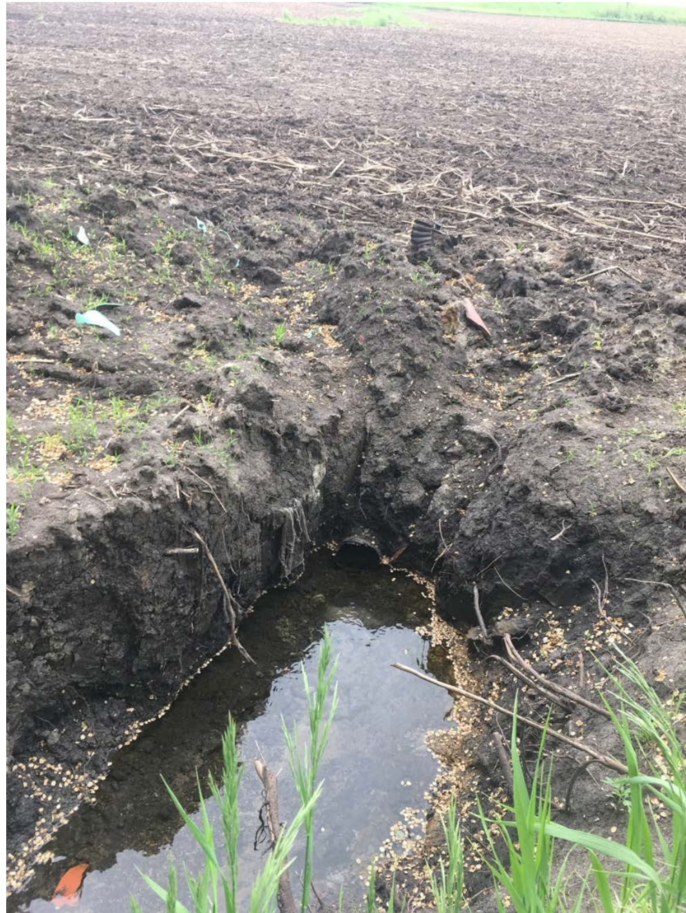
Figure 13. Tile drain outfall (center picture at water line) and associate gully erosion.
