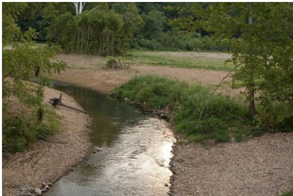
Photo 34. Sod matting on outside of a meander bend. Source: Stantec
