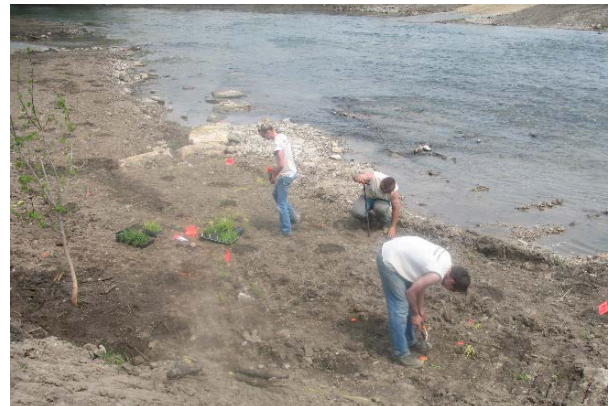
Photo 46. Planting vegetative plugs. Source: Iowa DNR
