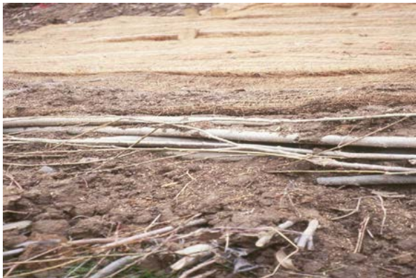
Photo 18. Installed fascine. Source: Stantec
