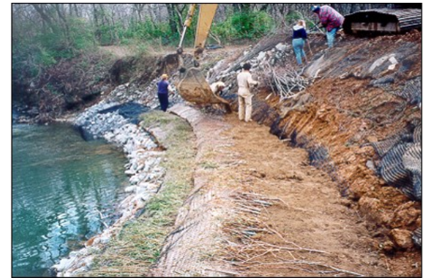
Photo 23. Bench excavation for brush layering. Source: Stantec
