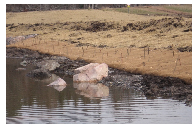
Photo 11. Live stakes in erosion control matting. Source: Collins & Baker Engineering
