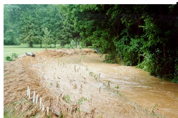
Photo 6. Live stakes in bankfull flow. Source: Charlotte-Mecklenburg Storm Water Services
