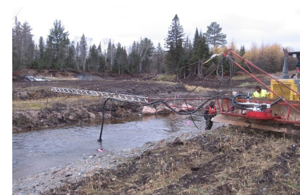
Photo 5. Hydraulic stinger live stake installation. Source: Lake Superior Tree Farm
