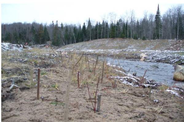
Photo 12. Live stakes installed in late autumn on Dead River, MI. Source: Collins & Baker Engineering
